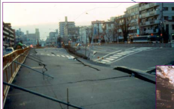
Kobe, 1995, Mw=6.9 Dakai subway
